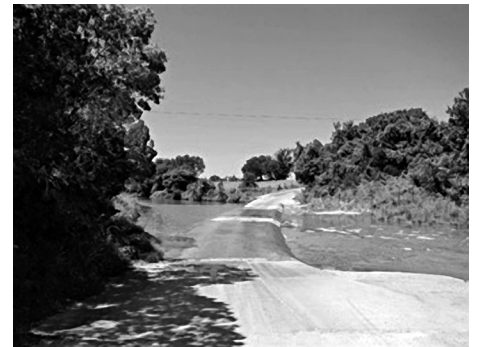
Low water crossing on the Paluxy River
